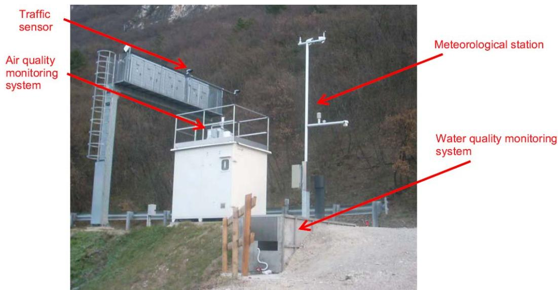
Figure 6: The first complete fixed monitoring site.
