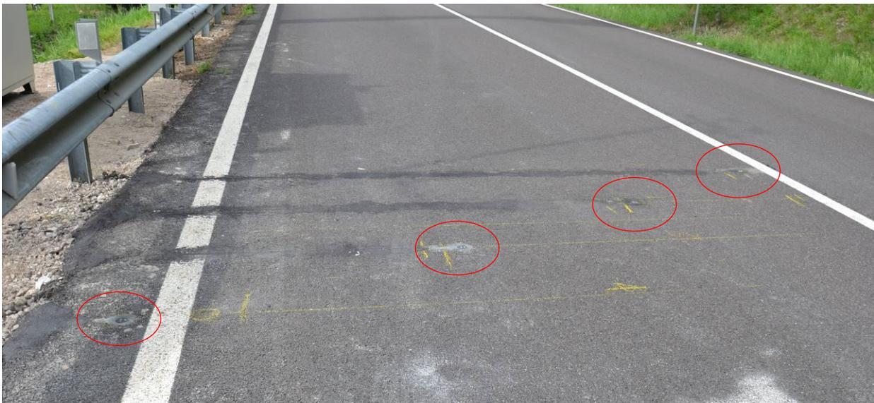
Figure 4: Sensors installed on the road surface
