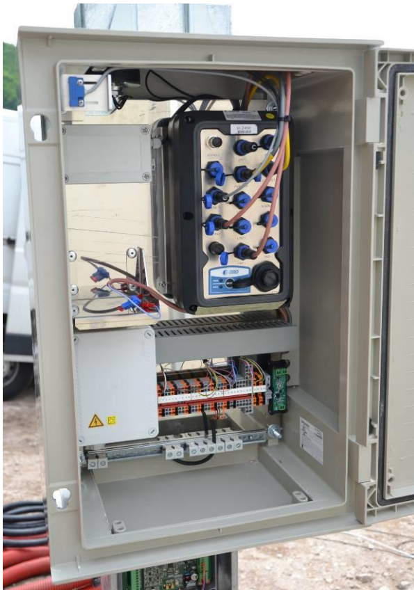
Figure 5: RWIS data management unit.
