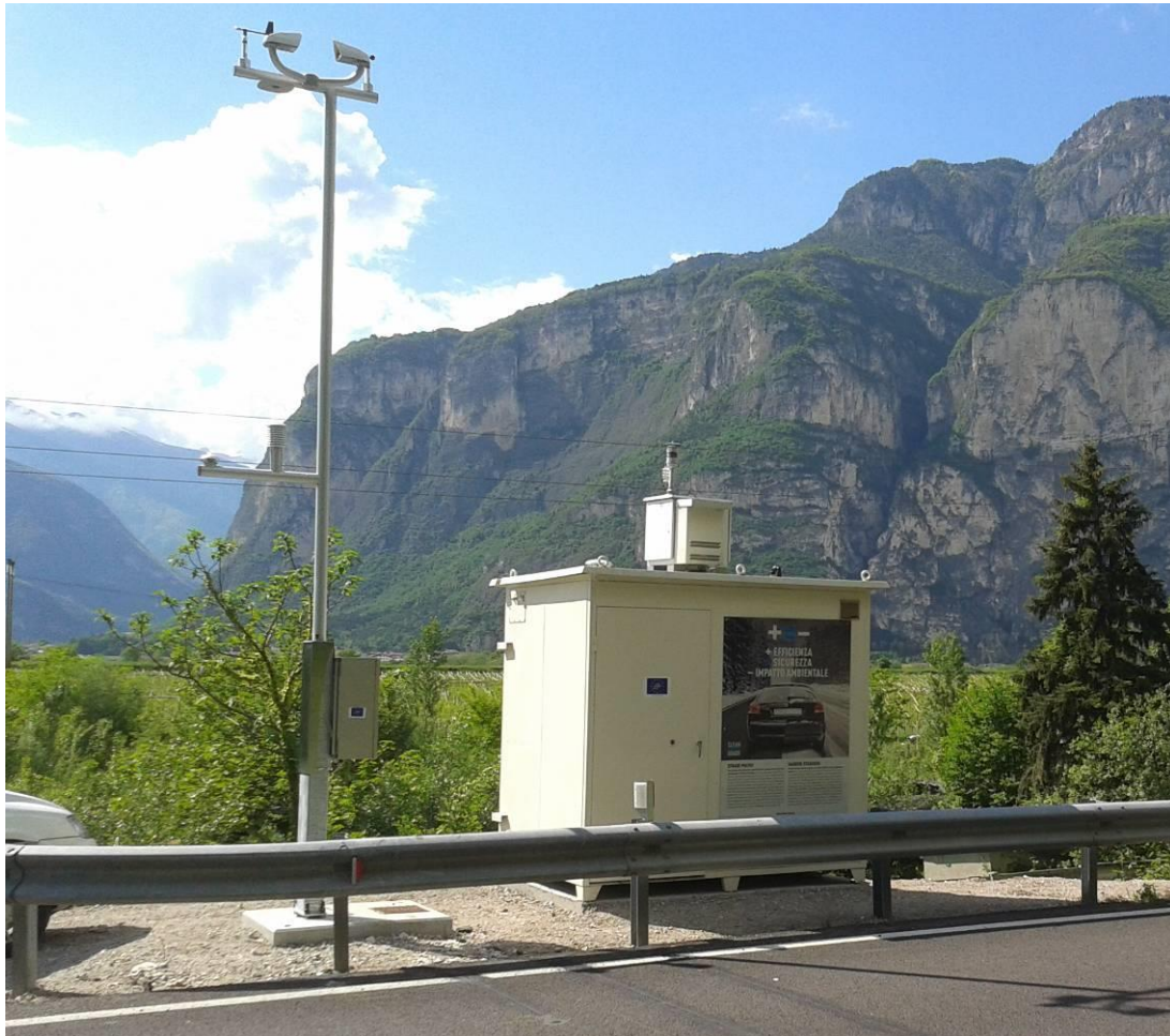
Figure 1: Typical configuration of RWIS station.
