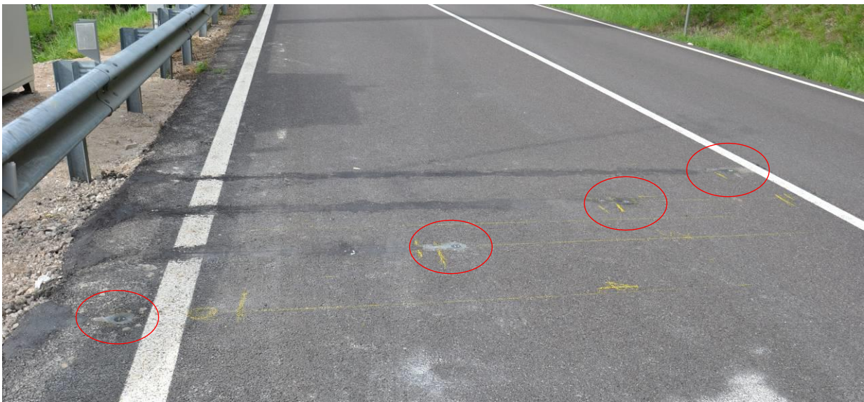
Figure 4: Sensors installed on the road surface
